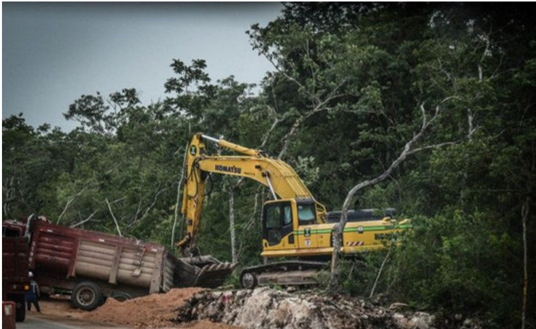
A heavy machine clears a path through the vegetation, felling trees during the construction of the Maya Train. Credit: Rafael del Río.
